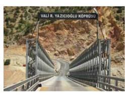
65+13m span of steel bridge 150 tons designed to erect as panel bridge. Bridge designed for cantilever launching. Single lane H20-S16 load rating. The bridge has been constructed as an economical alternative to conventional reinforced concrete bridges with shorter construction time. The low self-weight allowed low cost foundation at highly seismic and remote area. This bridge is the first panel bridge designed and manufactured in Turkey with span 67.5 meters.
